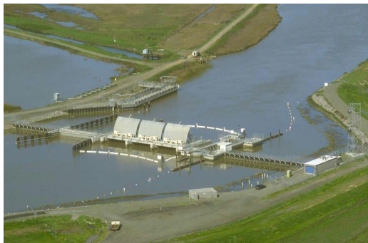
Salinity gates at Suisun Marsh (Credit: US Army Corps of Engineers)
